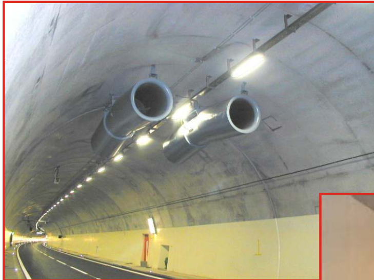
Uznaberg West Tunnel Switzerland
